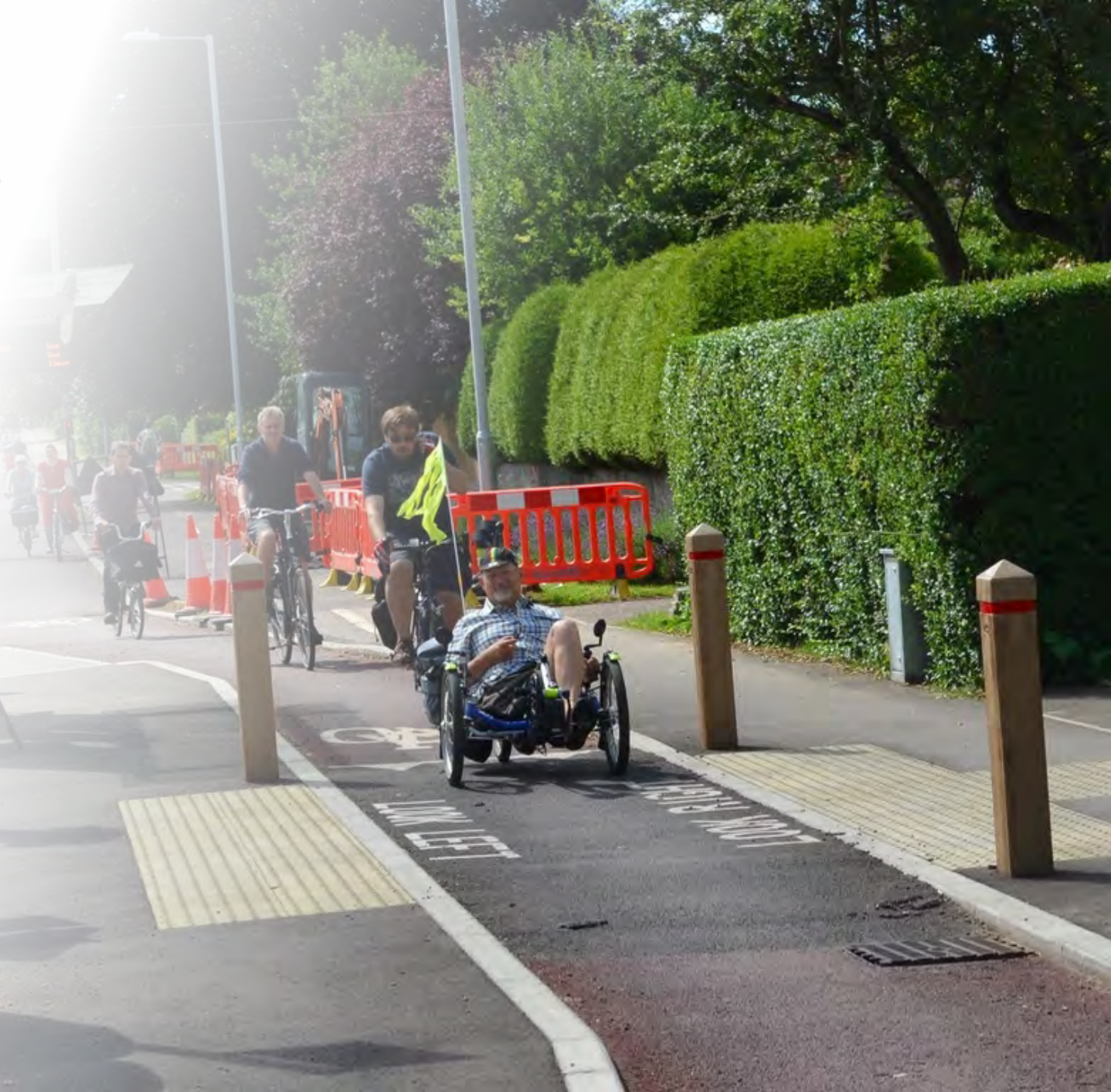
Image 37. Segregated cycle track and pedestrian crossing
