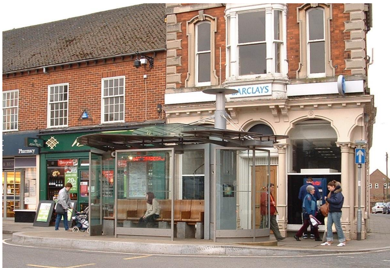
Figure 6-1 – Horncastle Interchange, Lincolnshire
